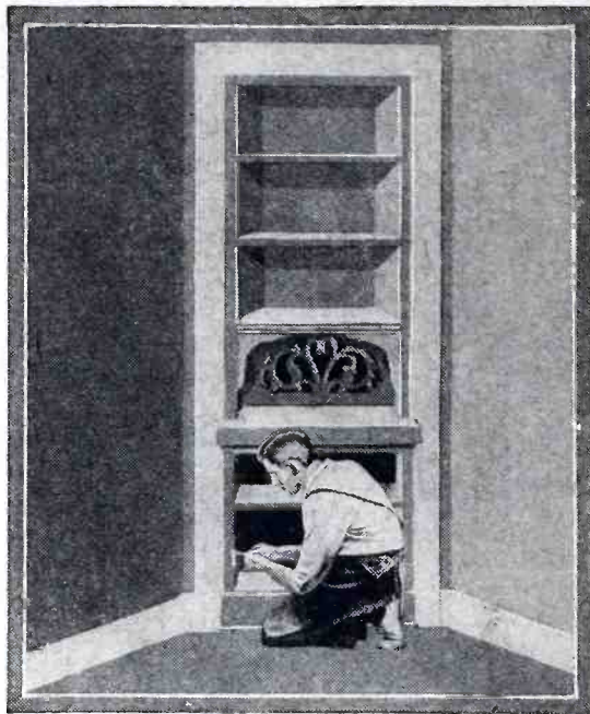
Fastening the hinges on the cabinet.
